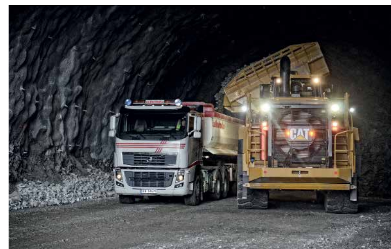
TUNNEL: Sidetipp forenkler tunnelling. (Foto: Pon Equipment)
